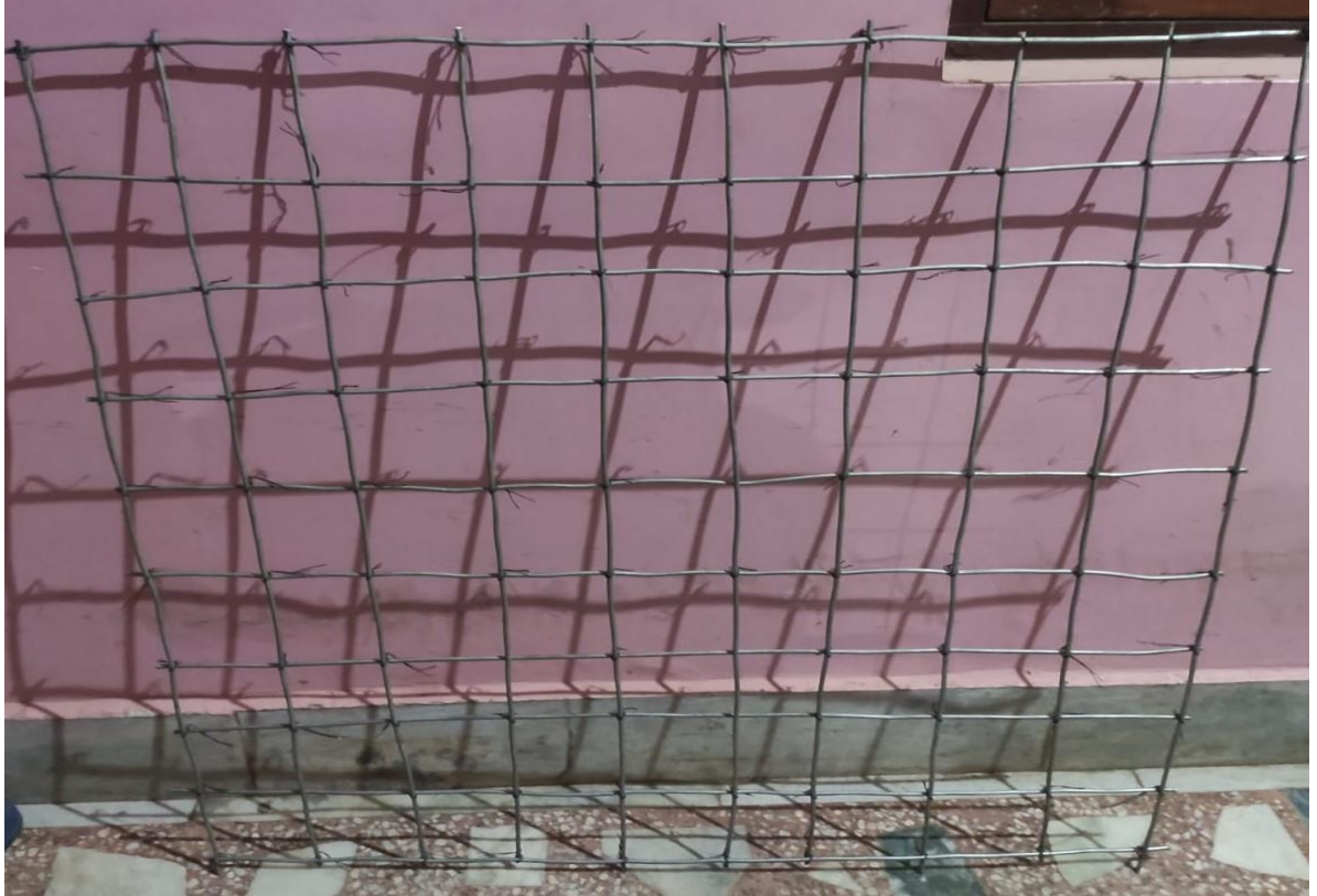
Figure 26: Winding of GI rod for slab fabrication
