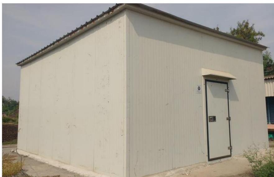
Fig 13: Controlled storage structure
