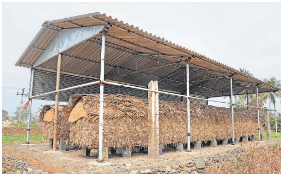
Fig 5: Roof over Pattarai
