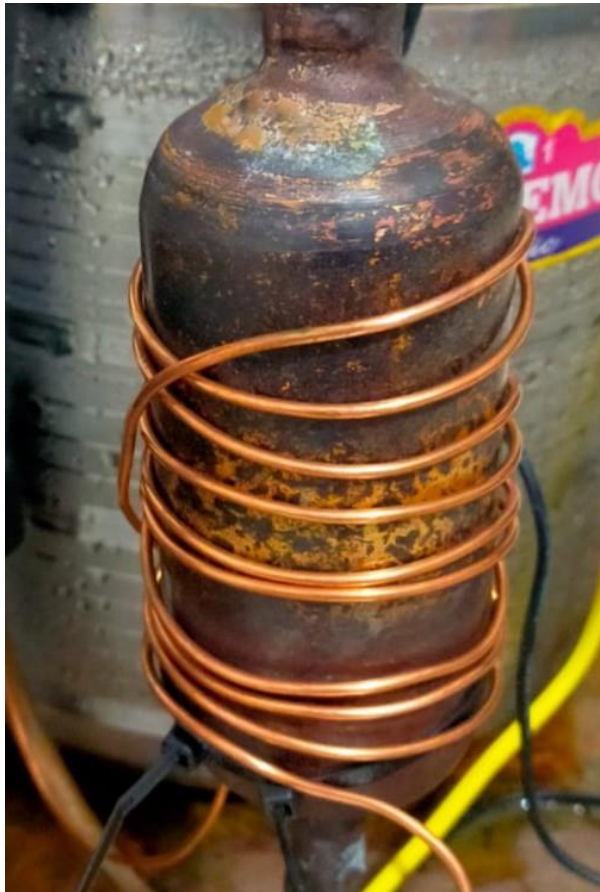
Fig.1.6 Accumulator and Capillary tube
