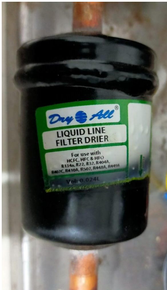
Fig.1.7 Filter Drier
